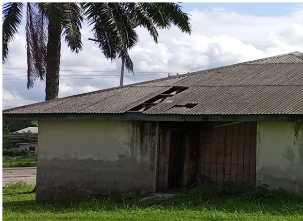
Figure 6b: A Building with Broken Asbestos Roof (Old Fashion) Source: Bazunu
